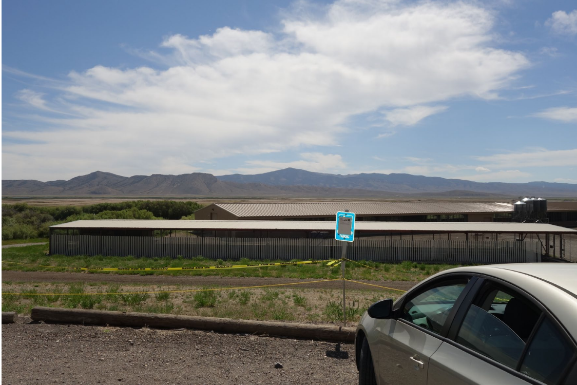
Gallagher Fish Hatchery Shade Shelter #1 – FCA Building #0936 Description: Exterior of the Structure.
