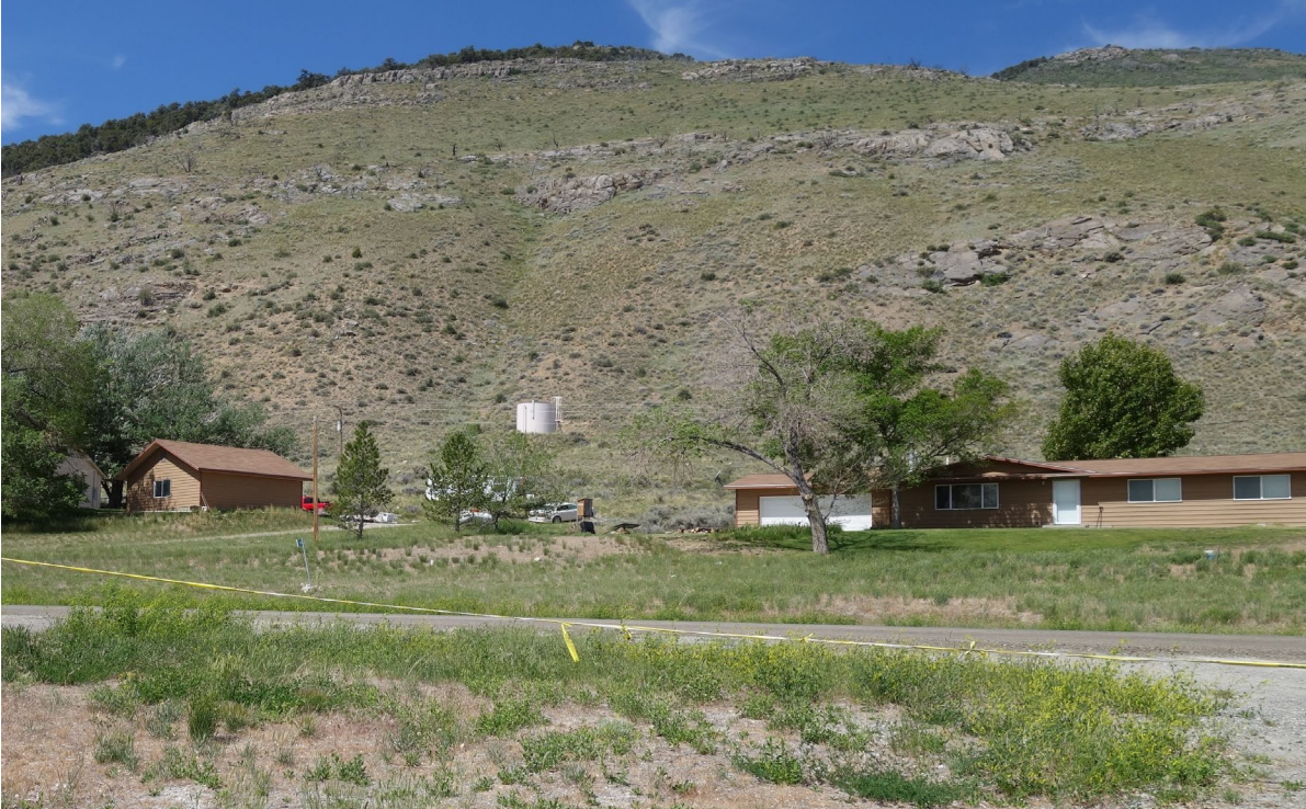
Water Tank – FCA Building #3139
