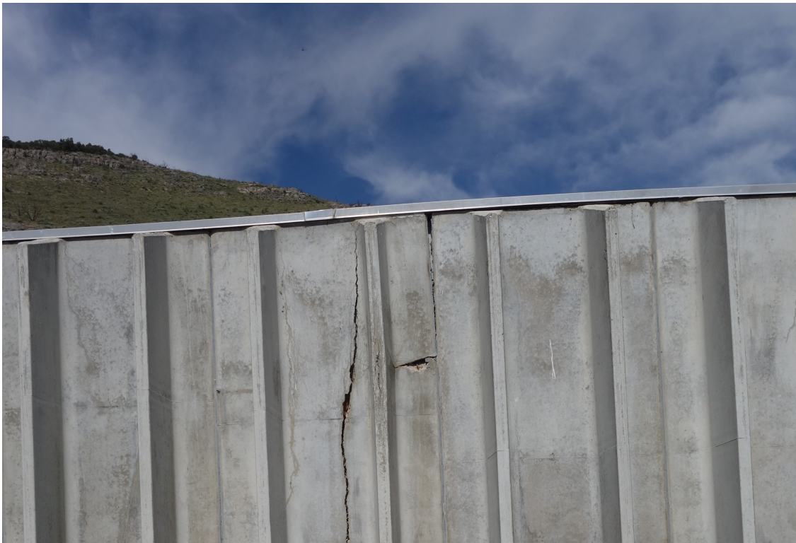
Gallagher Fish Hatchery – FCA Building #0922 Description: Building Structural Repairs.
