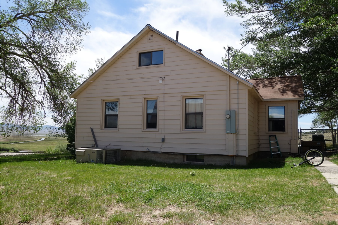
Gallagher Fish Hatchery Residence #1 – FCA Building #0926 Description: Exterior of the Building.
