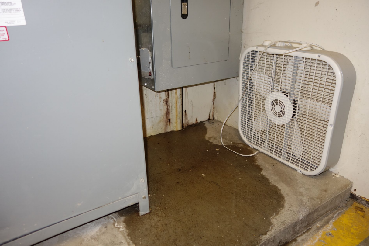
Gallagher Fish Hatchery – FCA Building #0922 Description: Water Intrusion Repairs.
