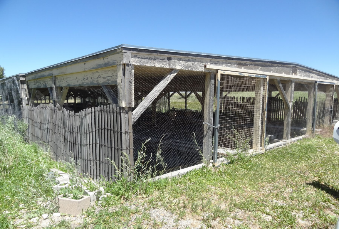
Gallagher Fish Hatchery Shade Shelter North – FCA Building #0935 Description: 2012 Photo - Demolish Structure Project Recommended.
