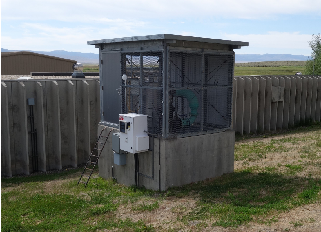
Control Box #1 – FCA Building #3143 Description: Exterior of the Building.
