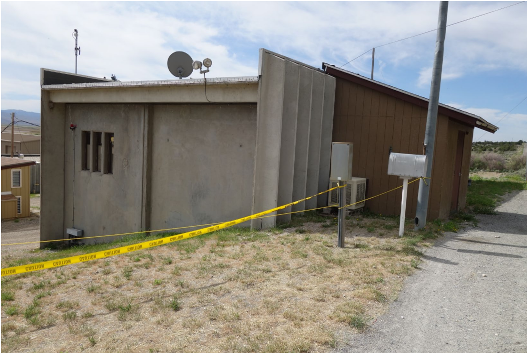
Gallagher Fish Hatchery Office & Shop – FCA Building #0923 Description: View of Main / Public Entrance.
