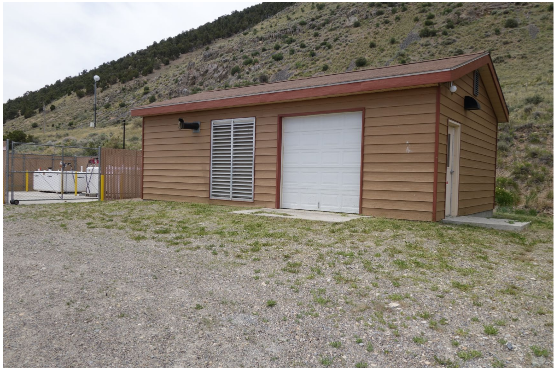
Emergency Generator Building – FCA Building #3142 Description: Exterior of the Building.
