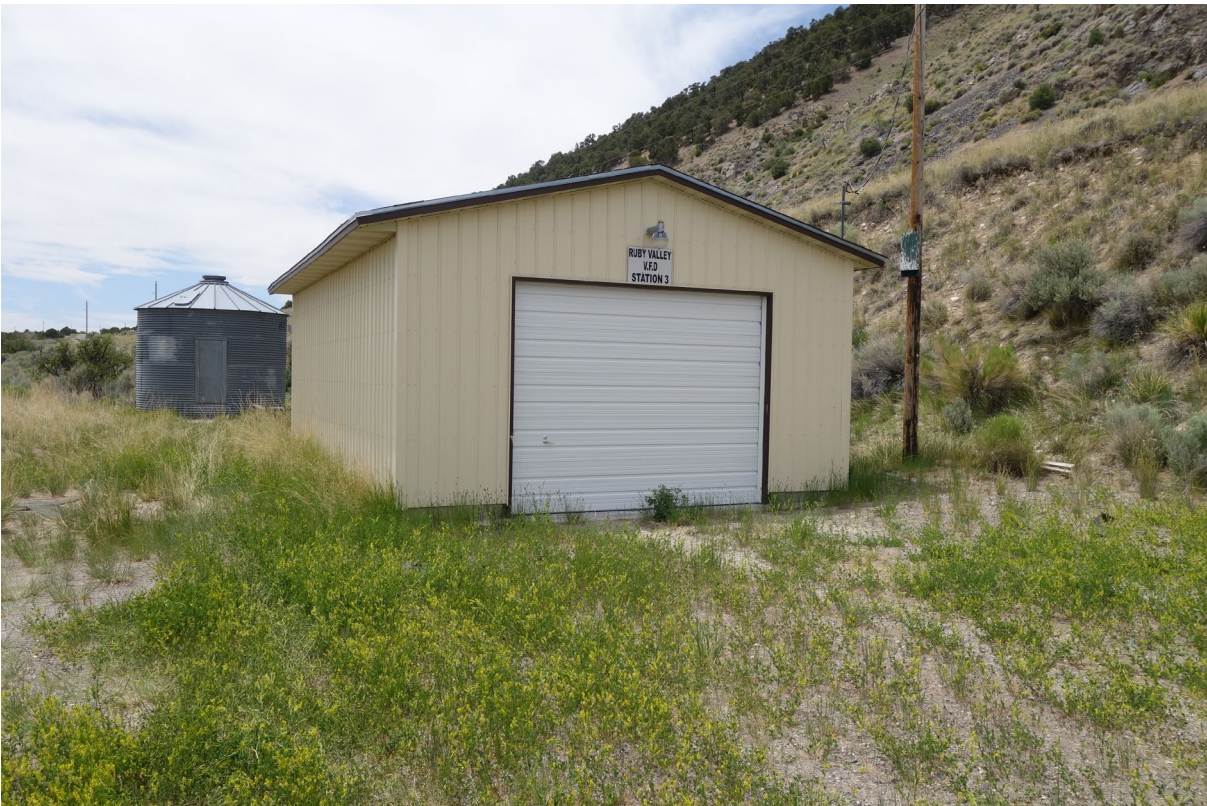
NDF Fire Truck Garage – FCA Building #2543
