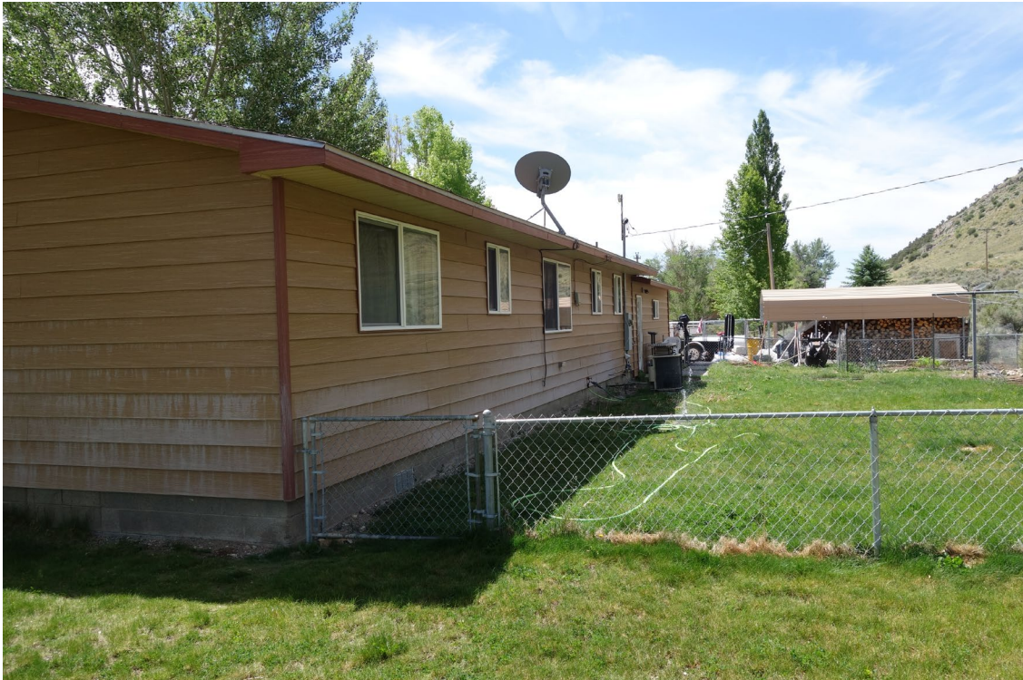
Gallagher Fish Hatchery Residence #6 – FCA Building #0934 Description: Exterior Finishes of the Building.
