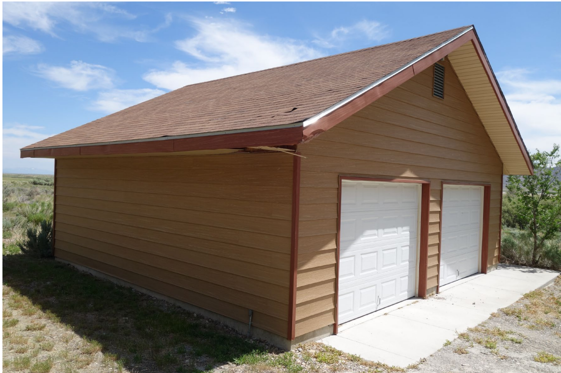
Residence #2 Garage – FCA Building #3146 Description: Structural Repairs Project.
