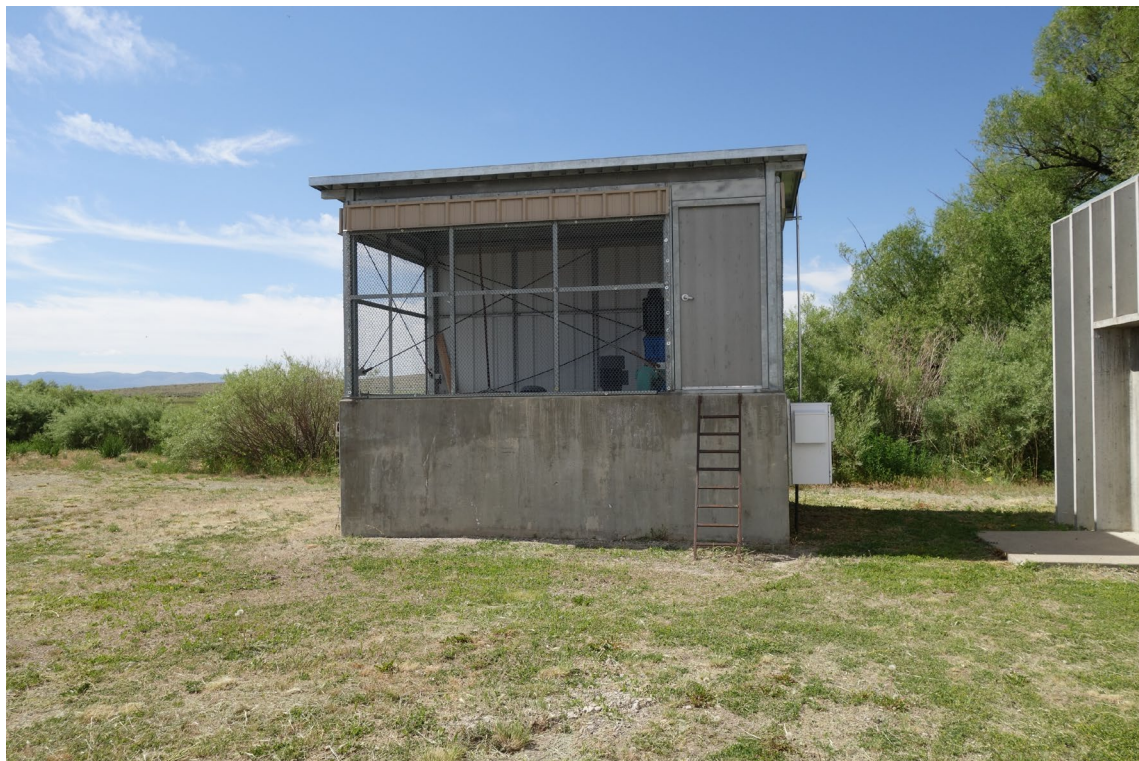
Control Box #2 – FCA Building #3144 Description: Exterior of the Building.
