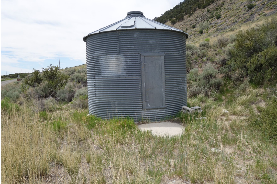
Metal Storage Building – FCA Building #2542 Description: Exterior of the Building.
