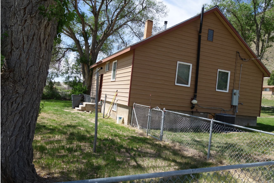
Gallagher Fish Hatchery Residence #2 – FCA Building #0928 Description: Exterior of the Building.
