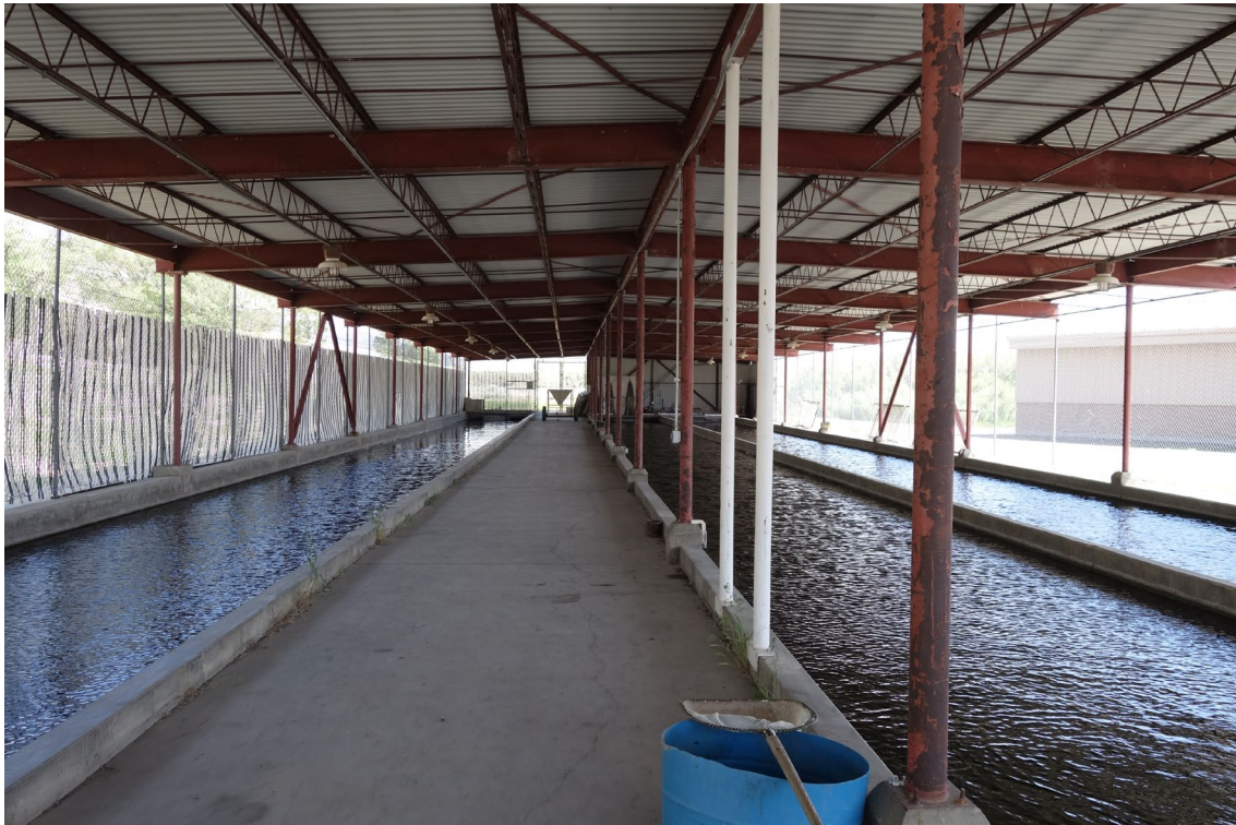
Gallagher Fish Hatchery Shade Shelter #1 – FCA Building #0936 Description: Interior Finishes of the Building.
