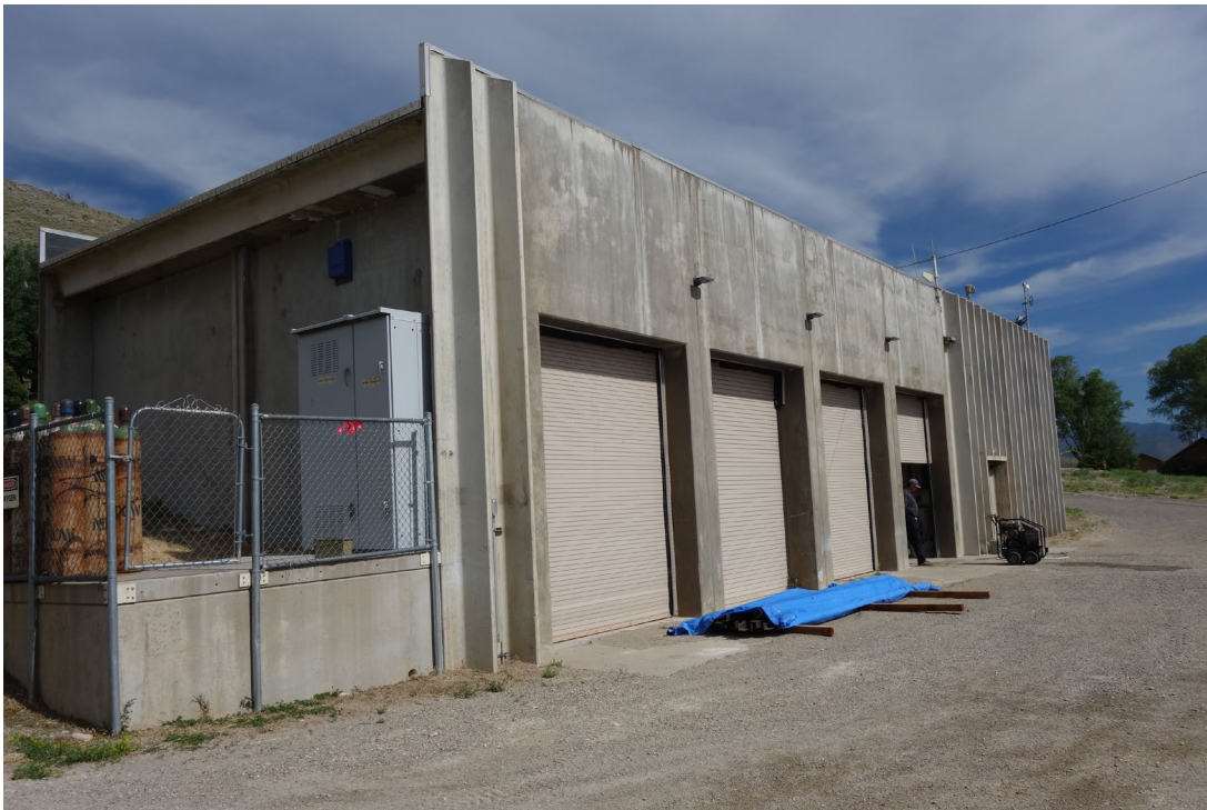
Gallagher Fish Hatchery Office & Shop – FCA Building #0923 Description: Exterior of the Building.
