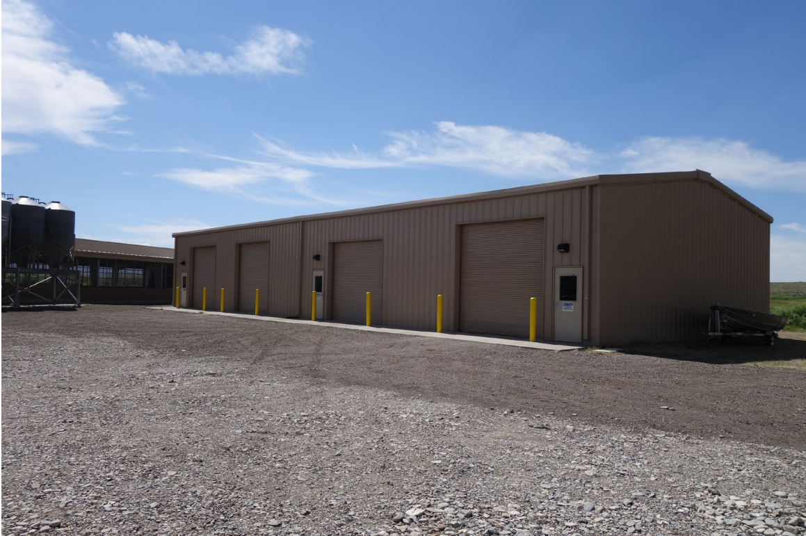
Vehicle Storage Building – FCA Building #3141 Description: Exterior of the Building.
