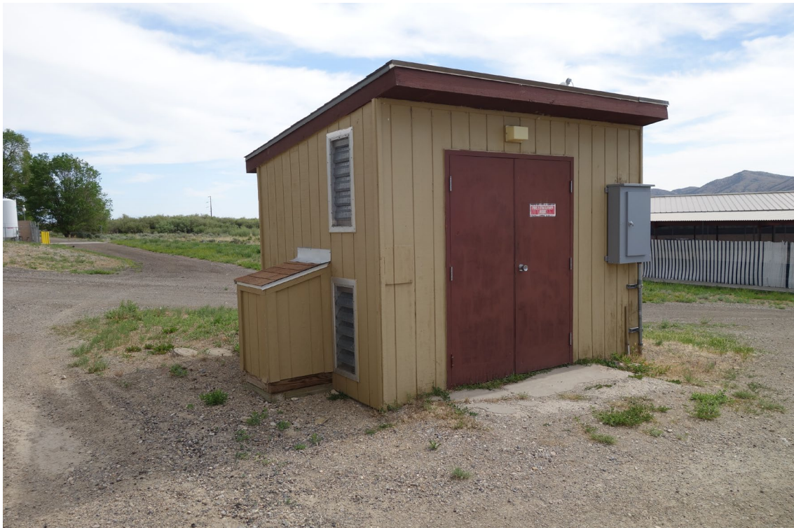
Domestic Pump House – FCA Building #0939 Description: Exterior of the Building.
