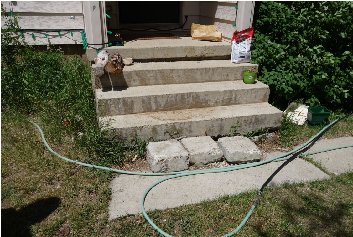
Gallagher Fish Hatchery Residence #1 – FCA Building #0926 Description: Concrete Stair Replacement & Handrail Installation.
