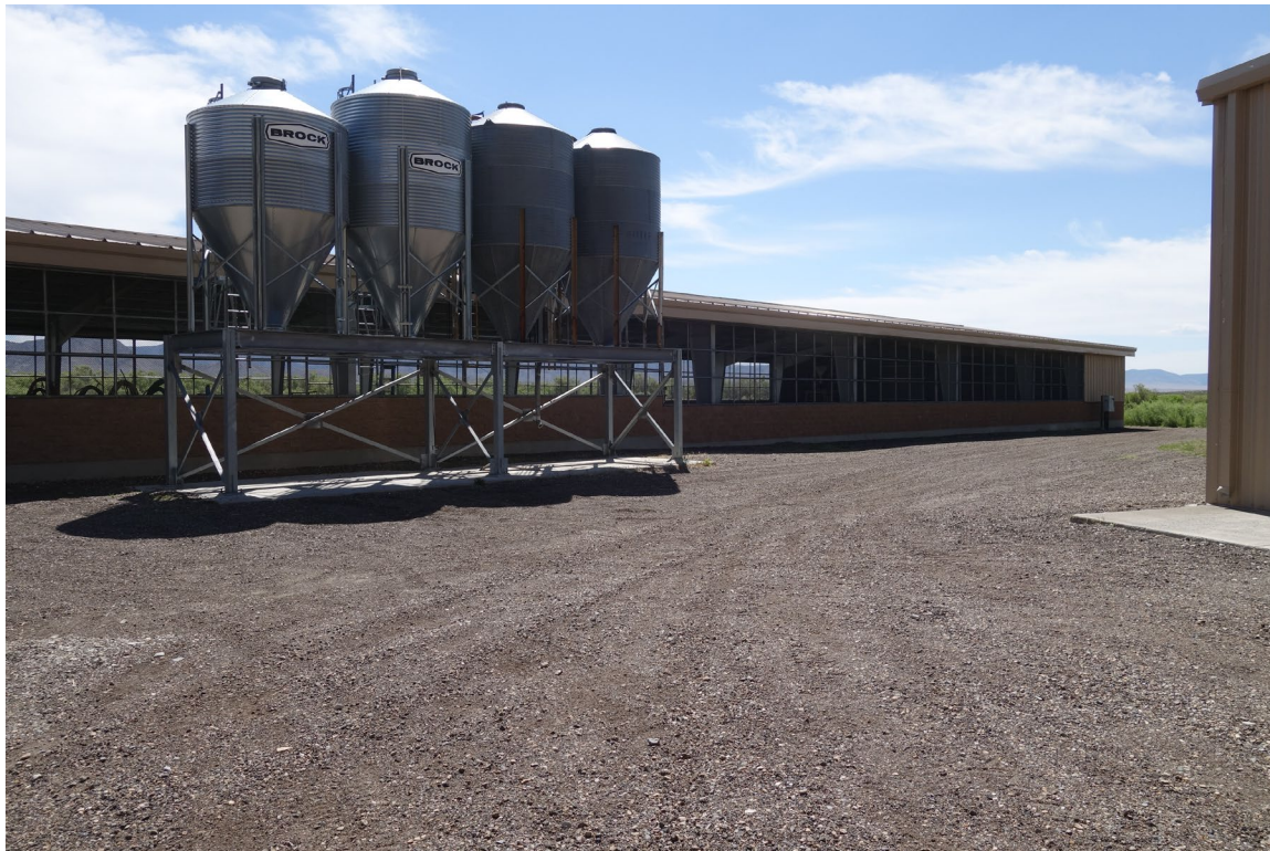
Rearing Building – FCA Building #3140 Description: Exterior of the Building.
