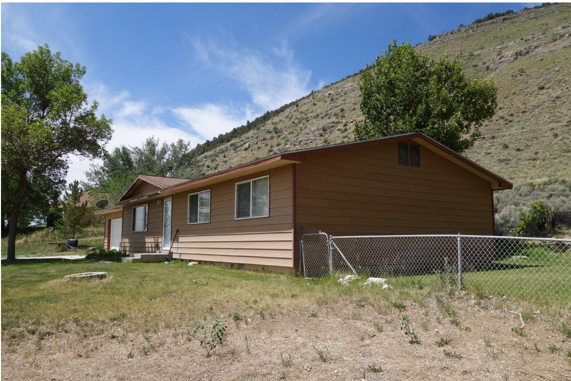
Gallagher Fish Hatchery Residence #4 – FCA Building #0932 Description: Exterior of the Building.
