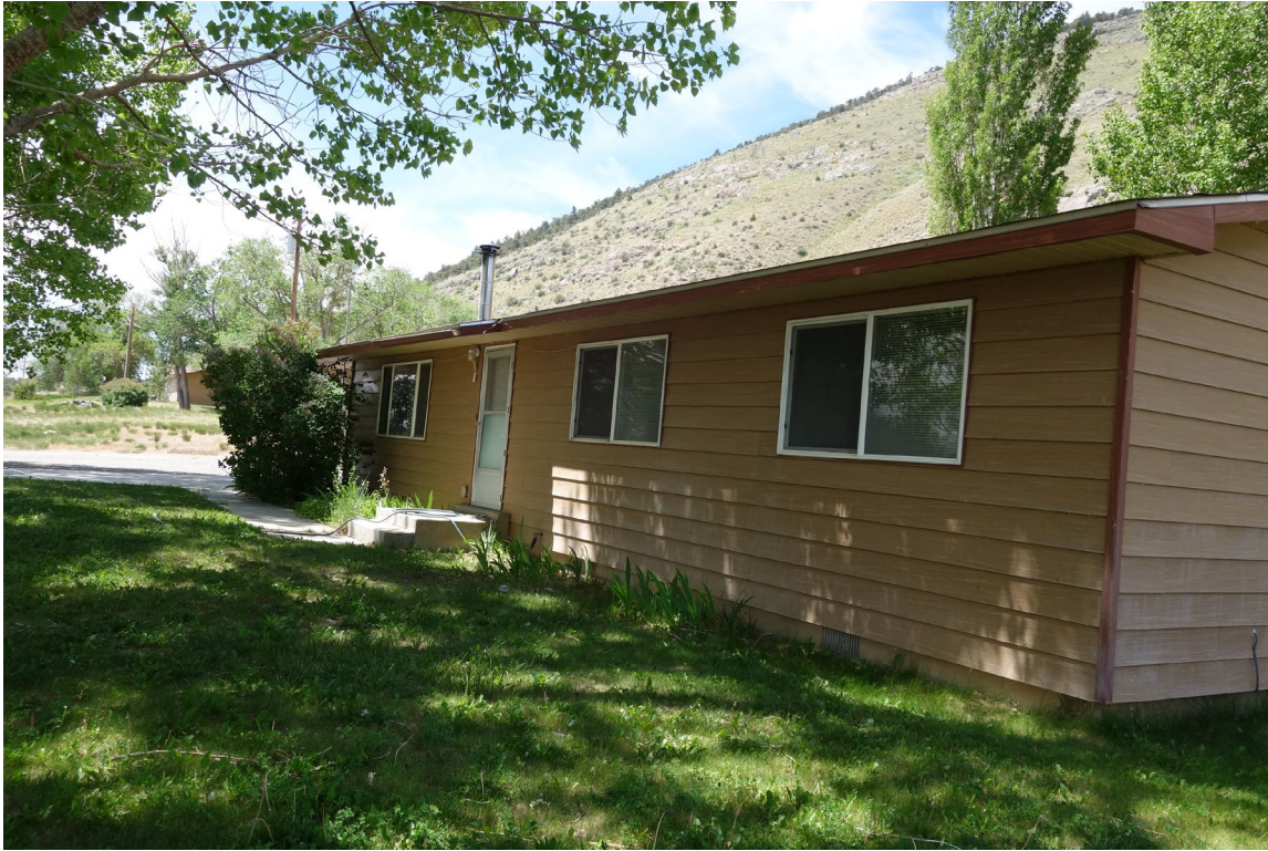
Gallagher Fish Hatchery Residence #5 – FCA Building #0933 Description: Exterior of the Building.
