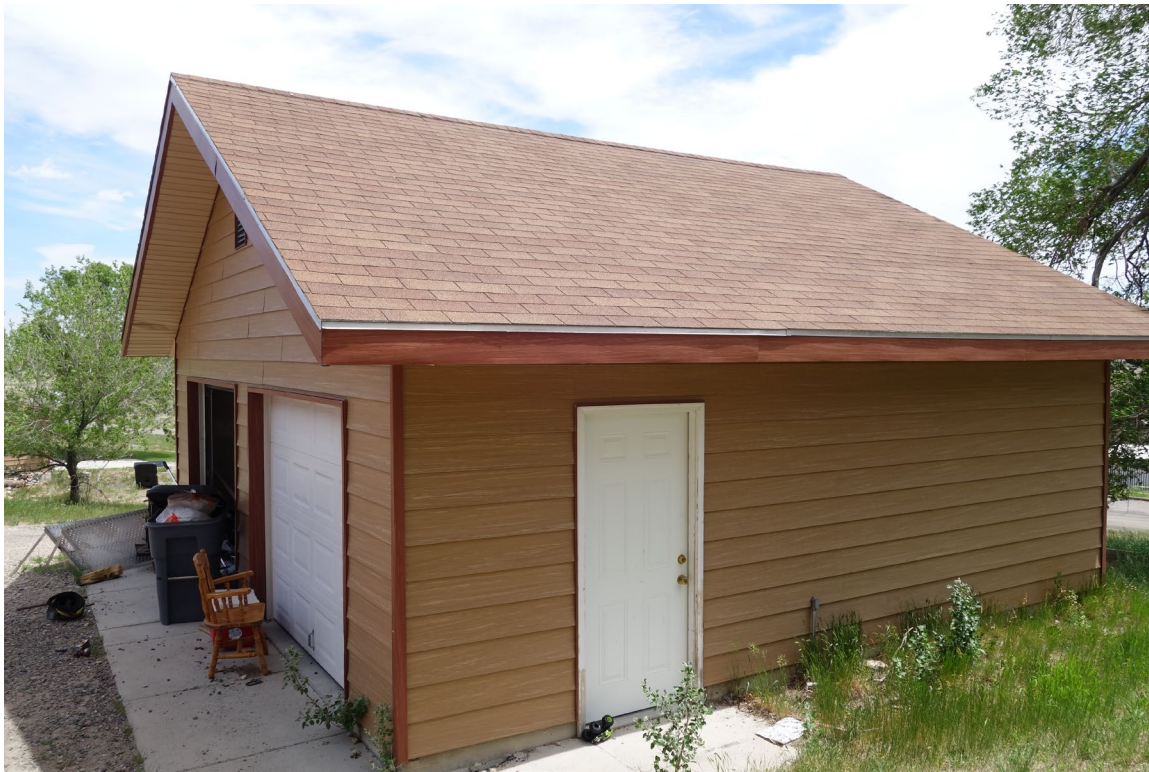
Residence #1 Garage – FCA Building #3145 Description: Exterior of the Building.
