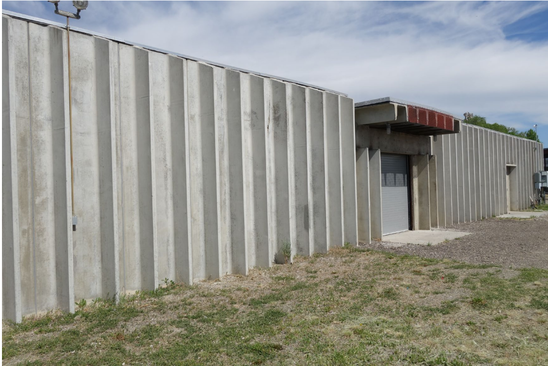
Gallagher Fish Hatchery – FCA Building #0922 Description: Exterior of the Building.
